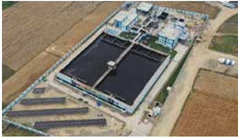
42+20+1 MLD Bareilly UP (includes solar plant)
