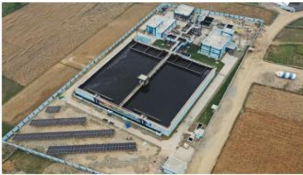
42+20+1 MLD Bareilly UP (includes solar plant)
