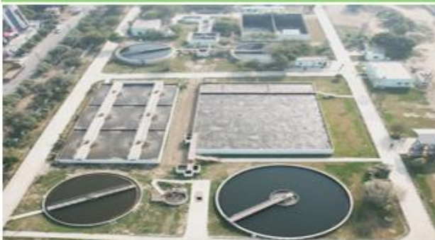
Upgradation of 5 MLD to 10 MLD CETP Rai Sonipat Haryana
