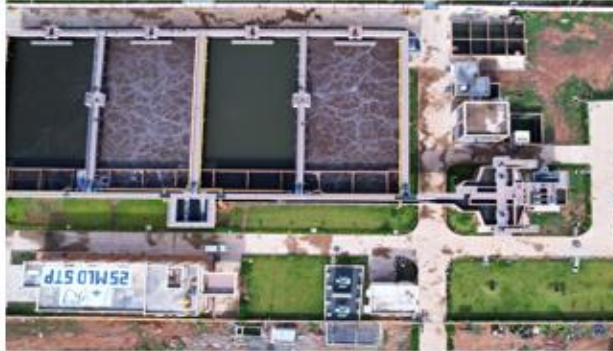
25 MLD STP Jagdalpur Chhattisgarh
