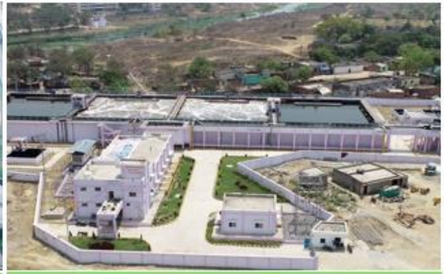
25 MLD STP at Raigarh Chhattisgarh
