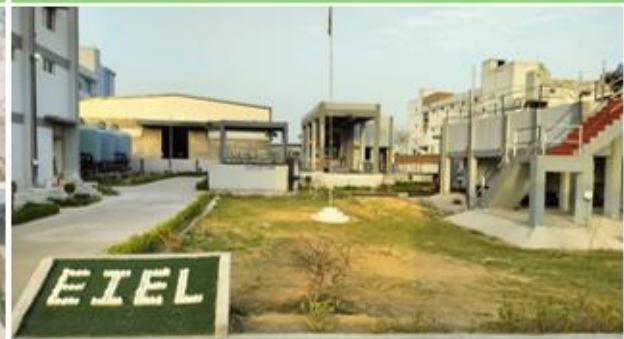
Upgradation of 16 to 26 MLD CETP Barhi Sonapat Haryana
