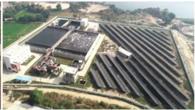
30 MLD STP Kota Rajasthan (includes solar plant)
