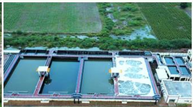
32.3 MLD STP at Surendernagar Gujarat
