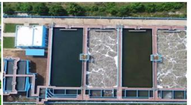
33 MLD STP Anand, Gujarat
