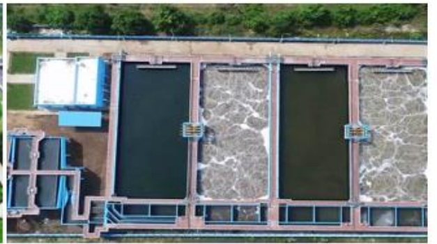
33 MLD STP Anand, Gujarat
