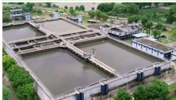
52 MLD STP at Bhatinda Punjab
