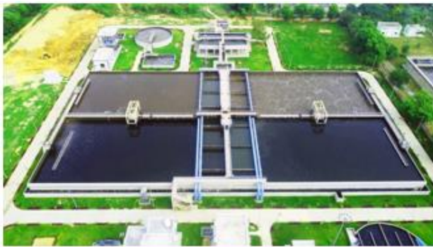
50 MLD STP Jalandhar Punjab
