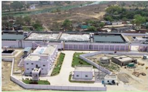
25 MLD STP at Raigarh Chhattisgarh
