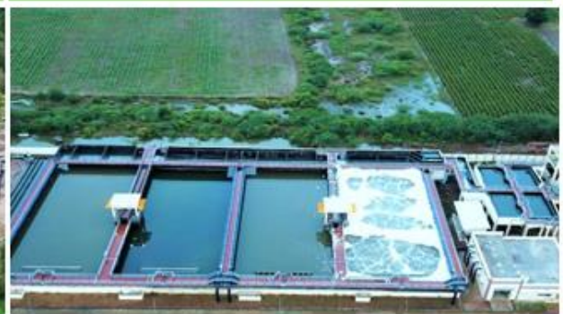
32.3 MLD STP at Surendernagar Gujarat
