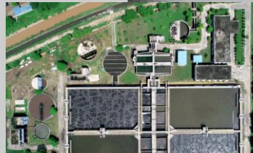
52 MLD STP, Bhatinda
